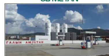
View of commissioned L-CNG fuelling station
